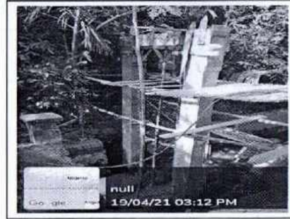
THANER KHAL LOCKGATE STRUCTURE
