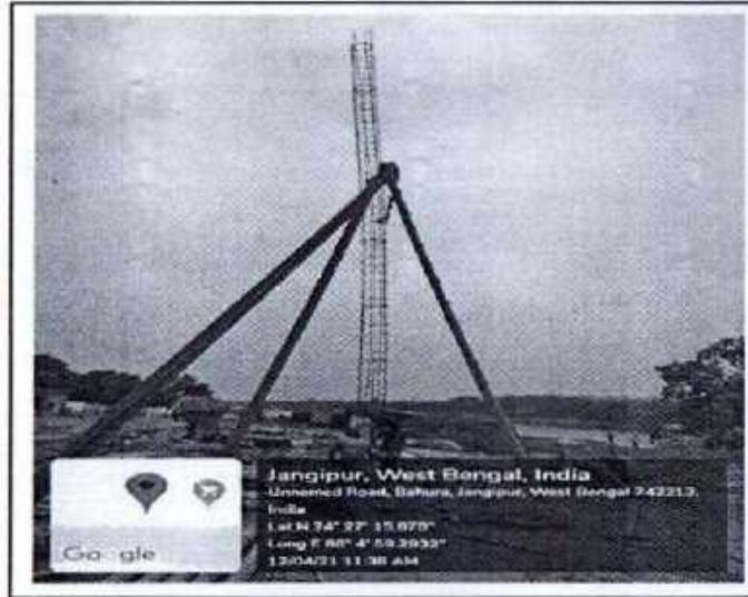
PILING WORK AT JANGIPUR STP SITE
