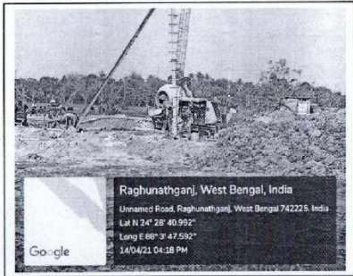
PILING WORK AT RAGHUNATHGANJ STP SITE
